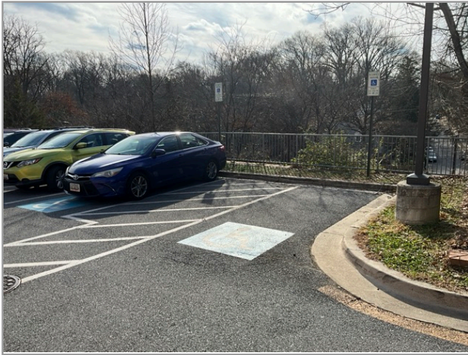
OVERVIEW OF ACCESSIBLE PARKING AREA
