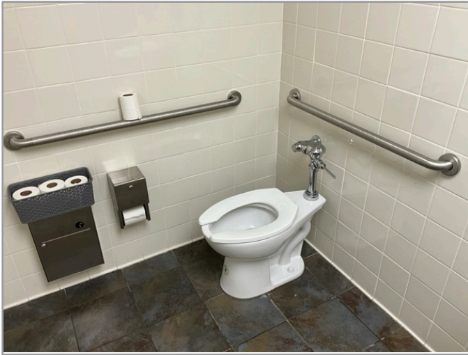
TOILET STALL OVERVIEW
