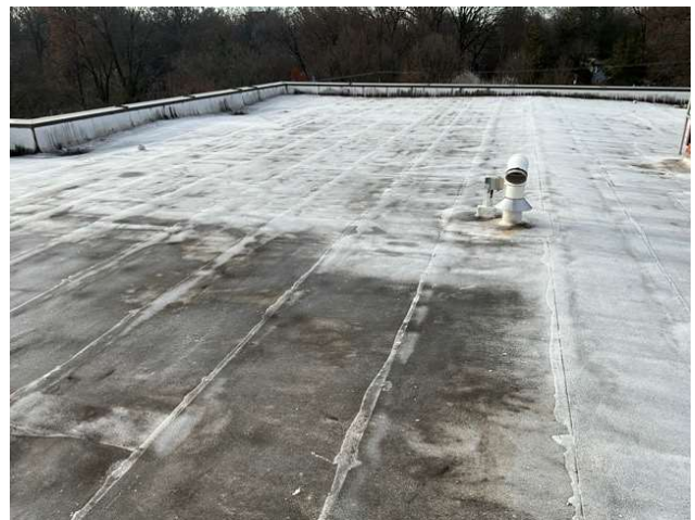
6 - MODIFIED BITUMEN ROOF
